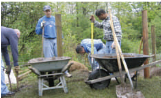
Volunteers doing trail stabilization work at MBG.
